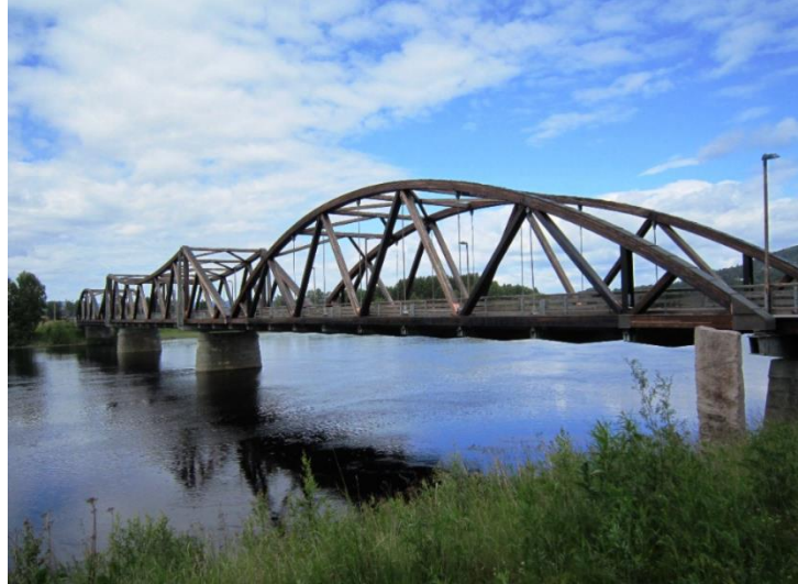
Figure 6.8: Flisa bridge, from https://structurae.net/en/structures/flisa-bridge
