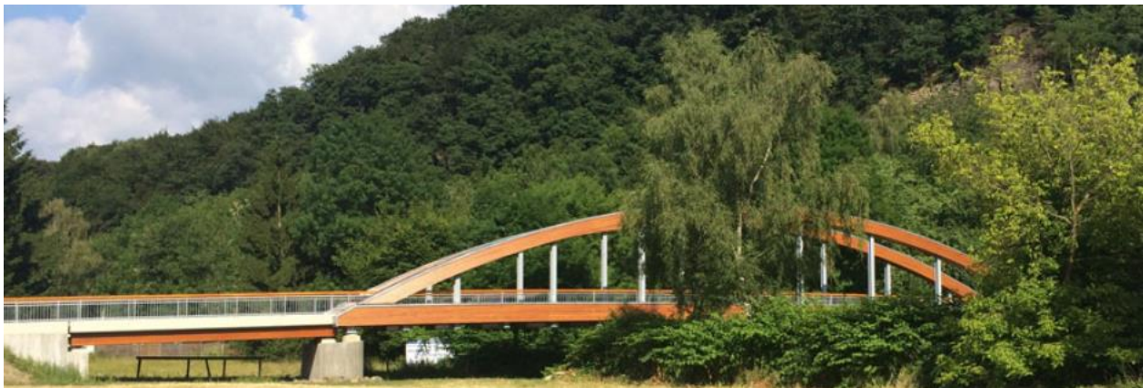
Figure 6.7: Lohmar Hengersberg bridge, from https://www.ib-miebach.de/en/projects/timber-bridges/arch-bridges-made-from-timber/long-span-timber-arch-bridge-hoengesberg-de.html
