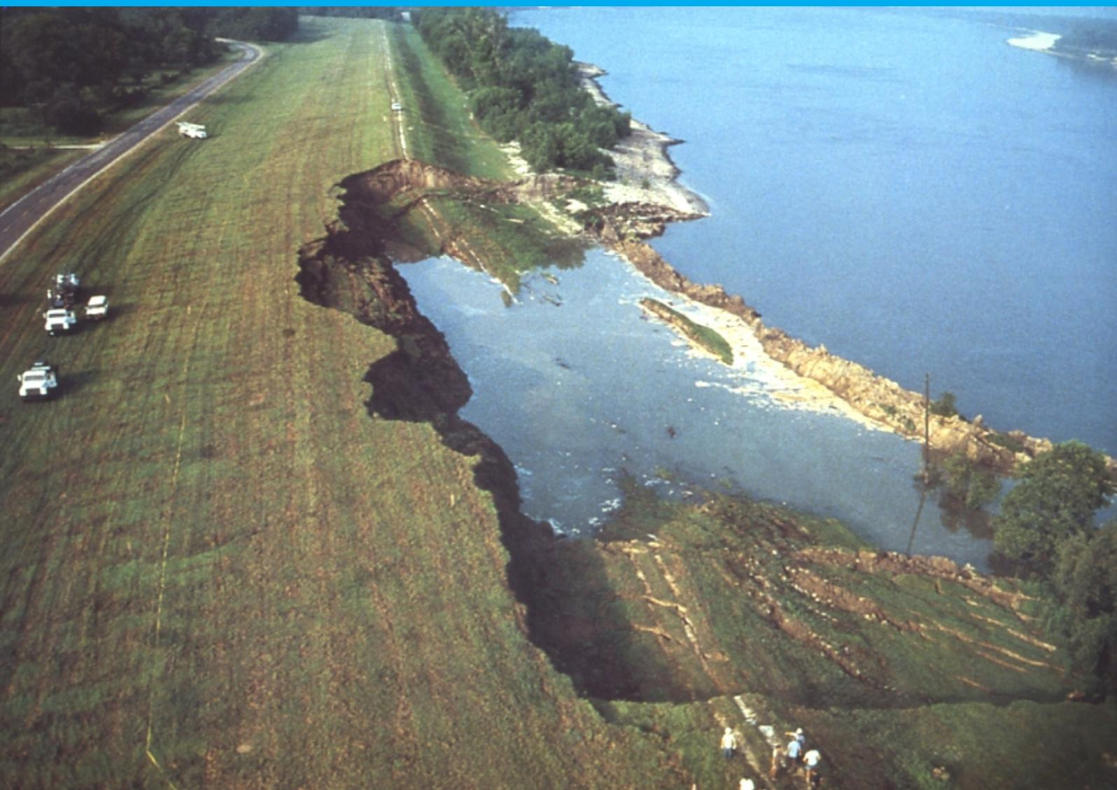
*Cover: Levee failure due to rapid draw down along the Mississippi River near Marchand, LA (Vanden Berge, 2014)*
