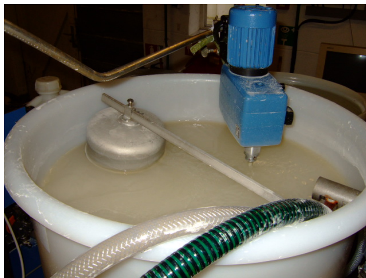
Figure 3.8 – water in the sludge softening vessel
