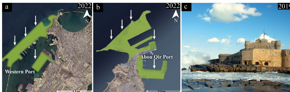
Figure 8. Mitigation procedures are currently being implemented in Alexandria: (a) beach nourishment supported by dikes and groynes in the western port and Abou Qir port, with areas of 176,000 m 2 and 56,655 m 2 , respectively. (c) In 2019, local authorities invested $14 million in dropping 4,700 concrete blocks around the historic fortress of the Gharb district to protect it from waves of coastal erosion. The figure was created using Adobe Photoshop (2019).
