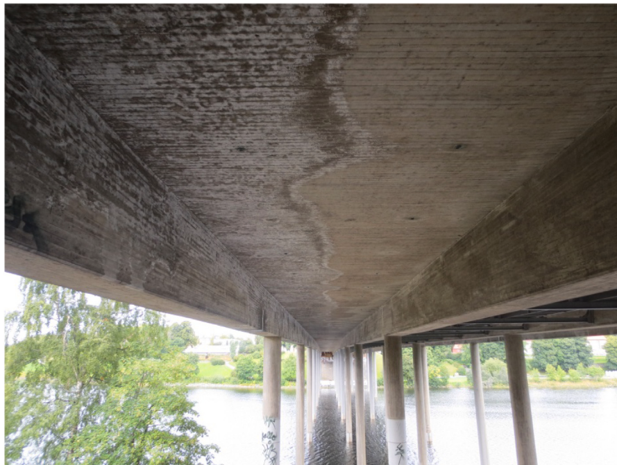
Fig. 7. There is a sign of water penetration of the bridge deck in outermost region of the bridge. The image shows the western outer and western inner beam. Image courtesy of Dr. Ing. A. Aas-Jakobsen AS.
