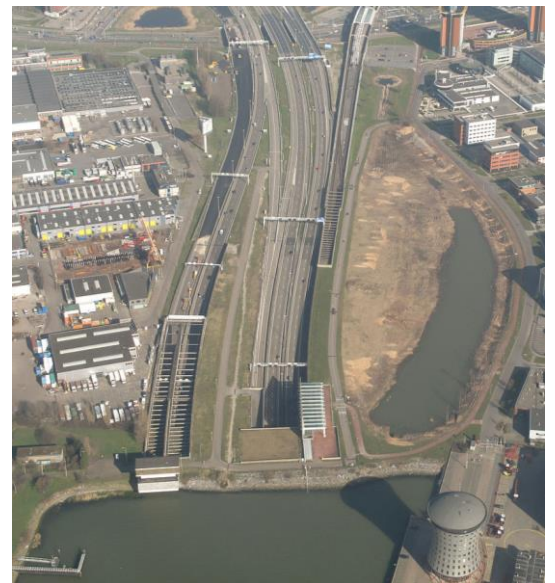
Figure 2.16: The access ramp on the Northern Bank [12]
