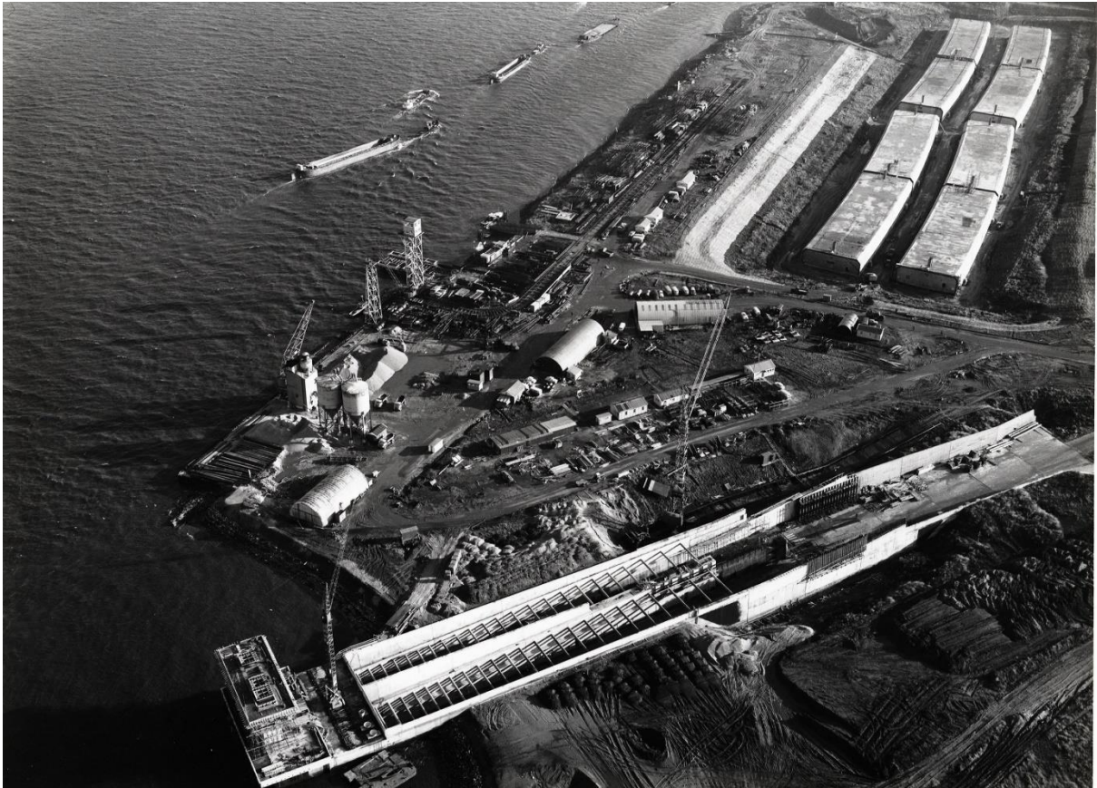
Figure 2.1: This image shows both the land part and the tunnel elements in the construction dock of the 1 st Beneluxtunnel [18]
