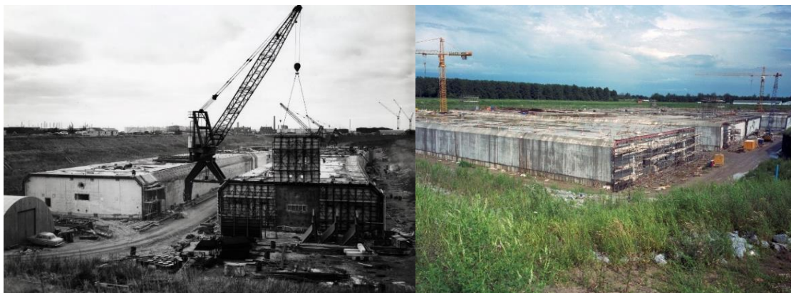
Figure 2.21: The elements of the 1 st (left) and the 2 nd (right) Beneluxtunnel during construction [26, 27]
