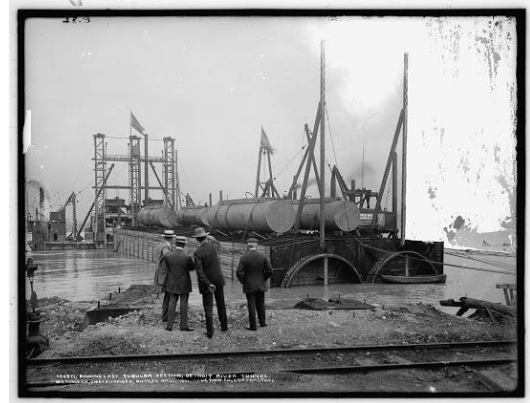
Figure 2.3: The Michigan Central Railway tunnel, completed in 1910 [2]
