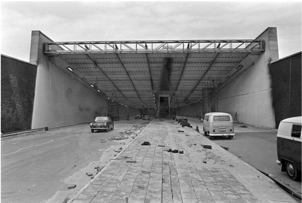
Figure 1.1: This image shows the 1 st Beneluxtunnel around the time when it was first introduced to the public. [16]
