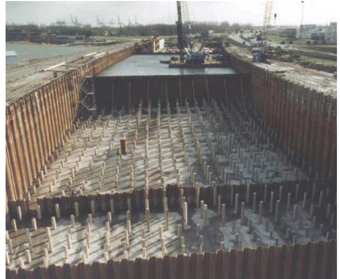
Figure 2.18: This figure shows the construction dock of the 2 nd Beneluxtunnel. It clearly shows the side walls, the underwater concrete floor and the tension piles.[7, 12, 13]
