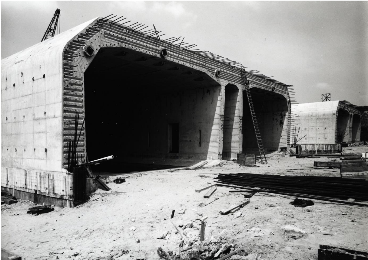
Figure 5.1: The tunnel elements of the 1 st Beneluxtunnel [12]
