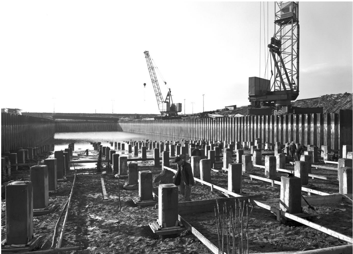
Figure 3.1: These foundation piles are the literal basis of the land parts of the 1 st Beneluxtunnel [40]
