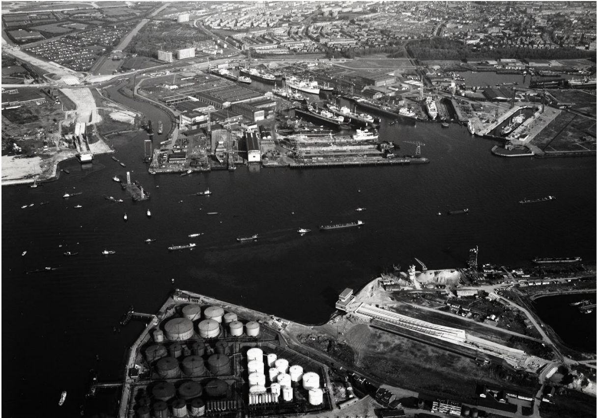
Figure 6.1: This image shows the construction of the 1st Benelux tunnel. The last element is being towed towards its desired position. [63]
