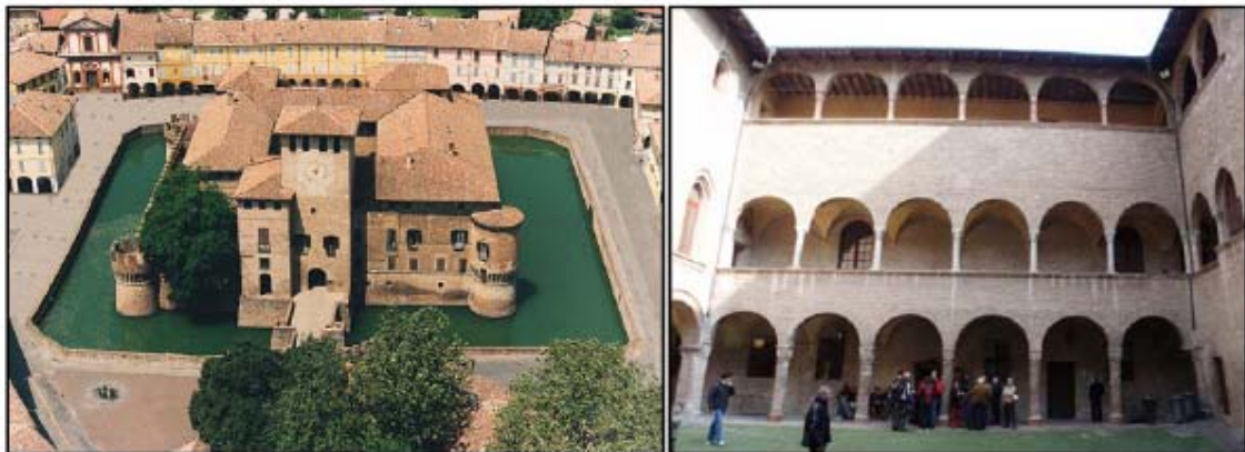
Figure 1: the Rocca di Fontanellato (left) and its "loggia" (right), whose columns need strenghtening.
