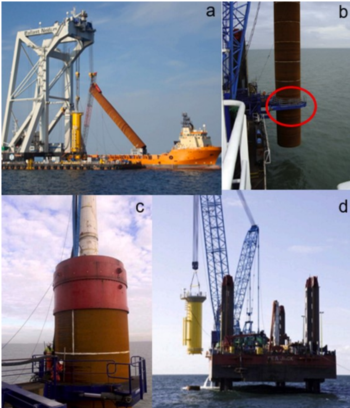
Figure 2.6: Monopile installation. a) Upending of the monopile from transportation barge. b) Gripper device (red circle) is used for positioning and handling of the monopile. c) Hydraulic hammer drives the monopile into the seabed. d) Grouting is used to cast the transition piece and monopile together.
