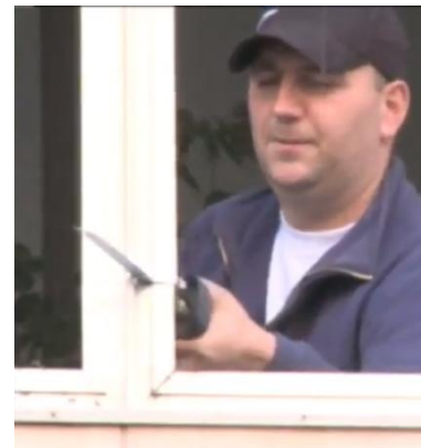
c. Saw-cutting aluminium profile
