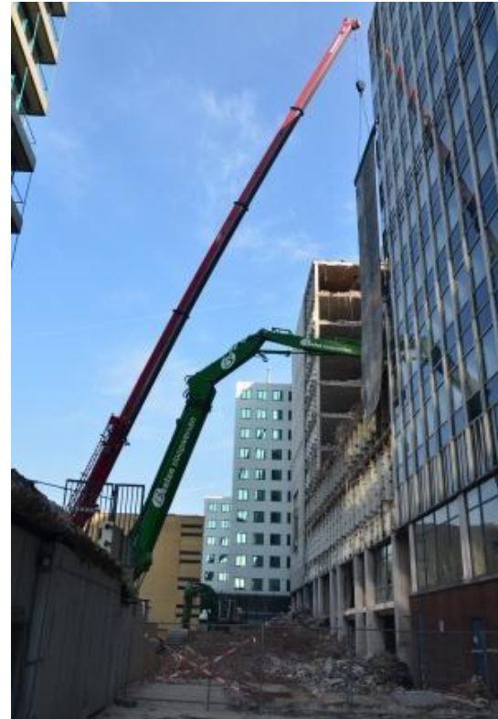
Figure 16 an example of application of the rubber membrane hung by a crane. Source: (Beelen-groep)
