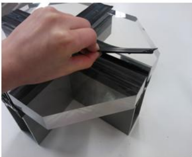
(1) Gasket -Glazing unit (2) Press fit (soft material) (3) Pull
