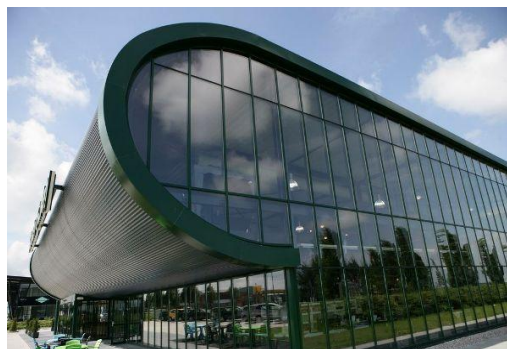
Figure 8 The research scope is limited in the standard type of glazed curtain wall system with aluminium profiles (Alcoa-architectuursystemen)
