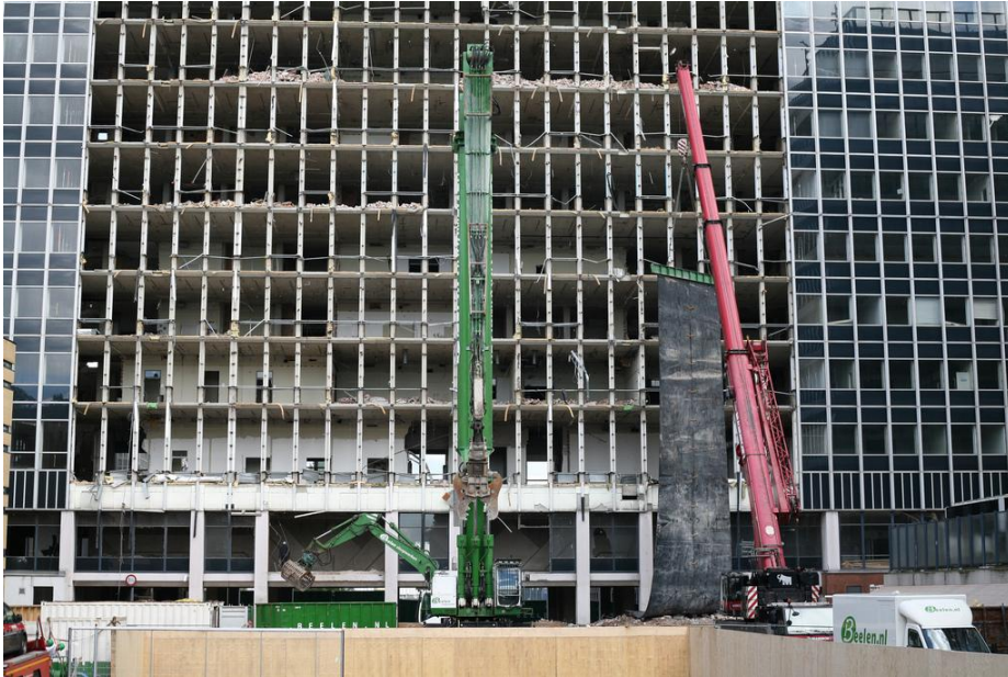
Figure 14 The University of Amsterdam (UVA) was striped out as a part of the renovation process. This project was delivered by BEELEN GROEP B.V
