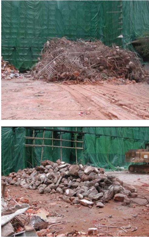
Figure 15 (top) Sorted steel stockpiled separately and (down) Sorted broken concrete stockpiled separately (Civil-Engineering-and-Development-Department, 2004)
