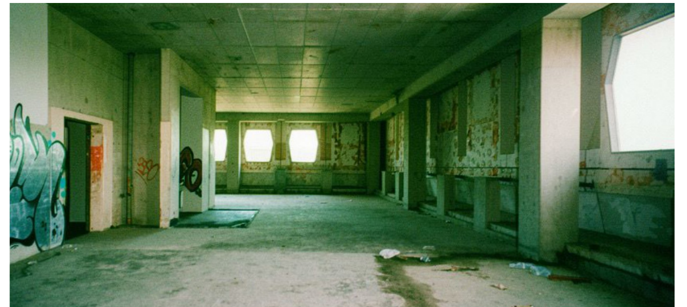
FIGURE 90: INTERIOR SITUATION OF THE TOWER
