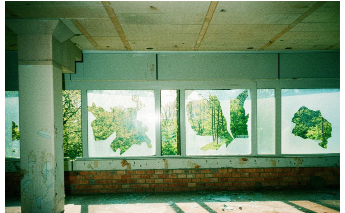
FIGURE 89: INTERIOR SITUATION OF THE BASE
