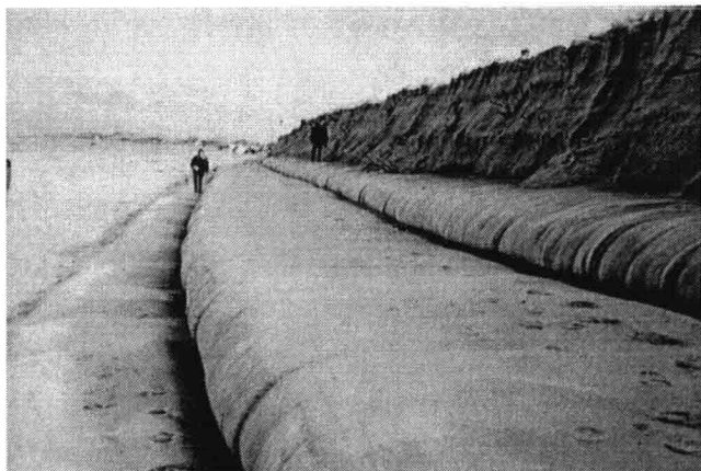
Fig. 11: Geotextile membrane combined with beach nourishment, Island of Sylt (from (13))
