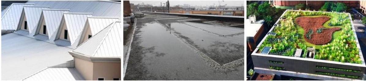
Figure 2.1: From left to right: a white roof with a high albedo value [37], a blue roof with water storage capacity [16] and an intensive green roof with a large diversity of vegetation types [21]
