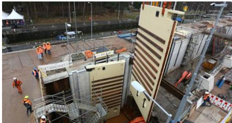
Figure 7: Installation of the composite lock gates [Photo courtesy of FiberCore Europe]
