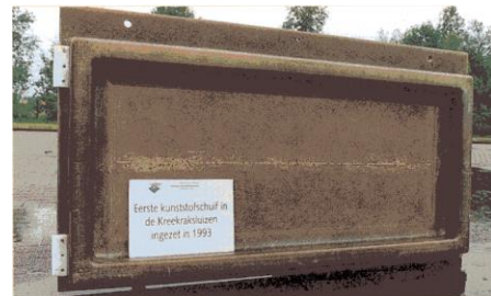
Figure 5: The first FRP gate of the Kreekraklock
