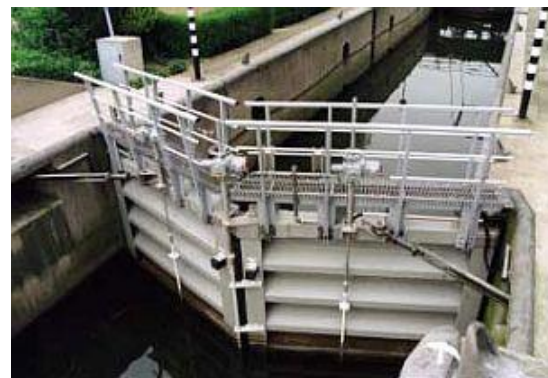
Figure 6: The FRP miter gates of the Spieringlock [Source: www.bhic.nl ]
