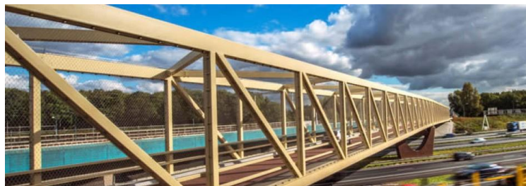
Figure 4: The hybrid overpass Nieuwe Houtenseweg at the A27
