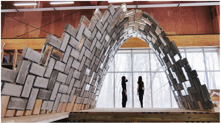
Figure 7: Prototype of assembled brick vault at Princeton University (Source: Parascho et al., 2021)
