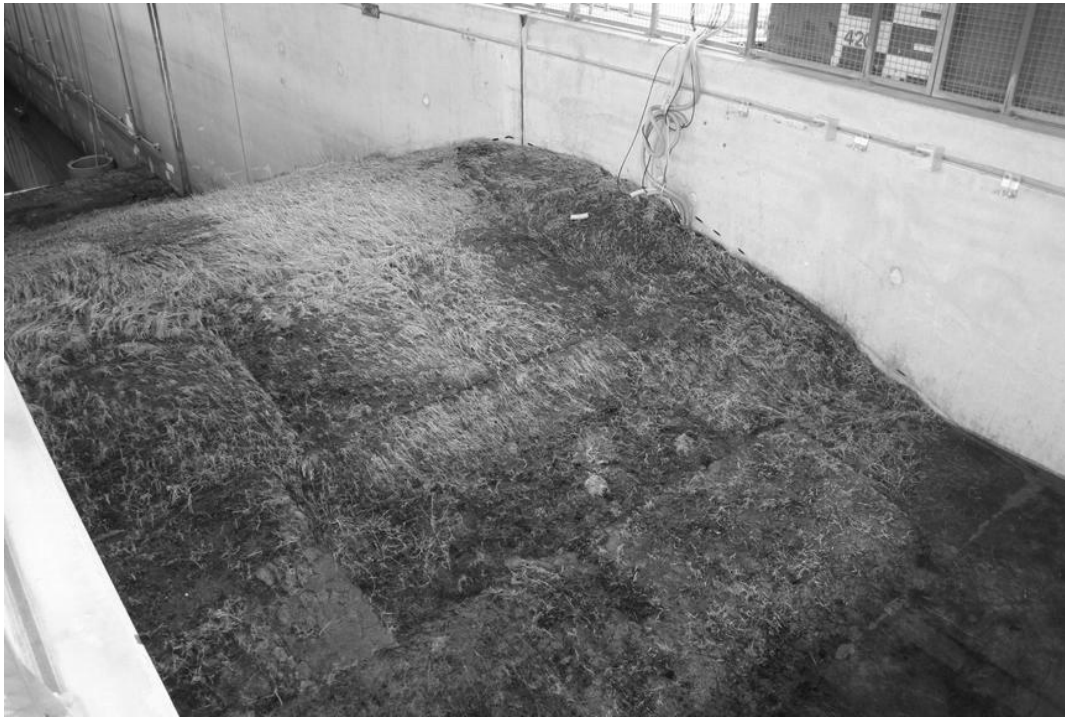
Figure 14. Flood-side grass cover during overtopping tests.
