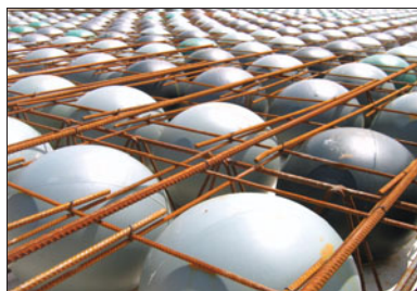
Figure 6-33 Example of a bubble deck slab
