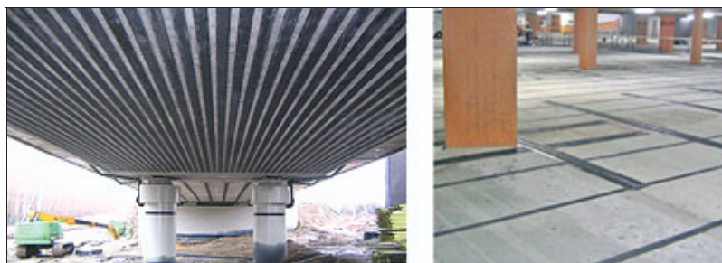
Figure 6-27 Application of carbon fibre lamellas
