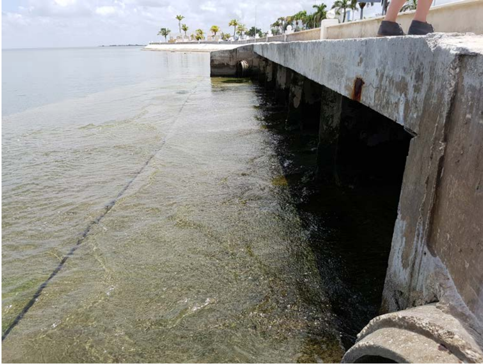
Figure G.3: Outlet of drainage system near Guadalupe
