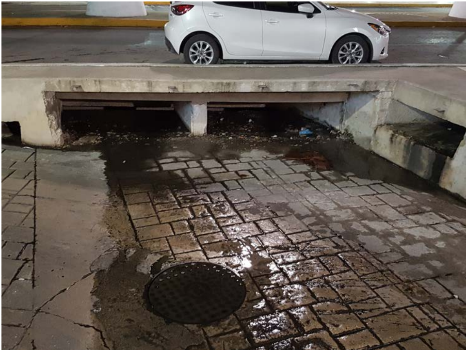
Figure G.6: Inlet of drainage system at the end of Calle 14
