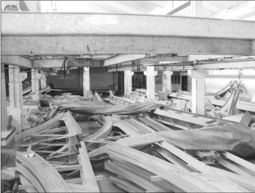
5. Elements of the hall of the former Gare du Sud, removed and stored in Nice.
