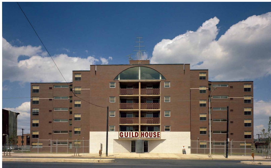
FIG. 2.14 Robert Venturi (Venturi and Rauch), Guild House, Philadelphia, Pennsylvania (1963). Front elevation. The Venturi's Guild House illustrates the metamorphic vocation of the architectural elements. An architectural element such as a window could grow in size to cover the full extension of the façade, and include the connective spaces of the building, therefore losing its original definition to acquire a new functional status.
