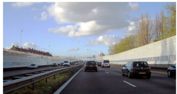
Fig. 7. Perspex screen and houses along the highway A13 close to Delft. (photo M.M.Minderhoud)
