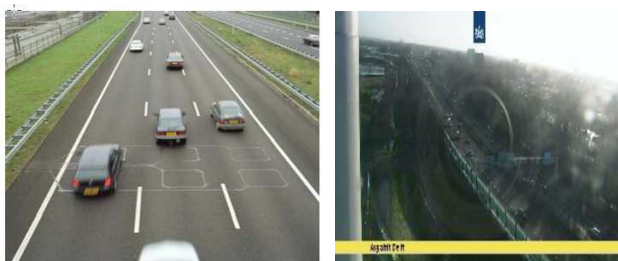
Fig. 9. Wires in the surface of roads and cameras along highway (photo Regiolab-Delft).
