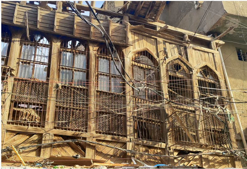
Figure 37. The neglect of shanashil work, made in palm wood (Source: photograph by Mohammed J. for the author).
