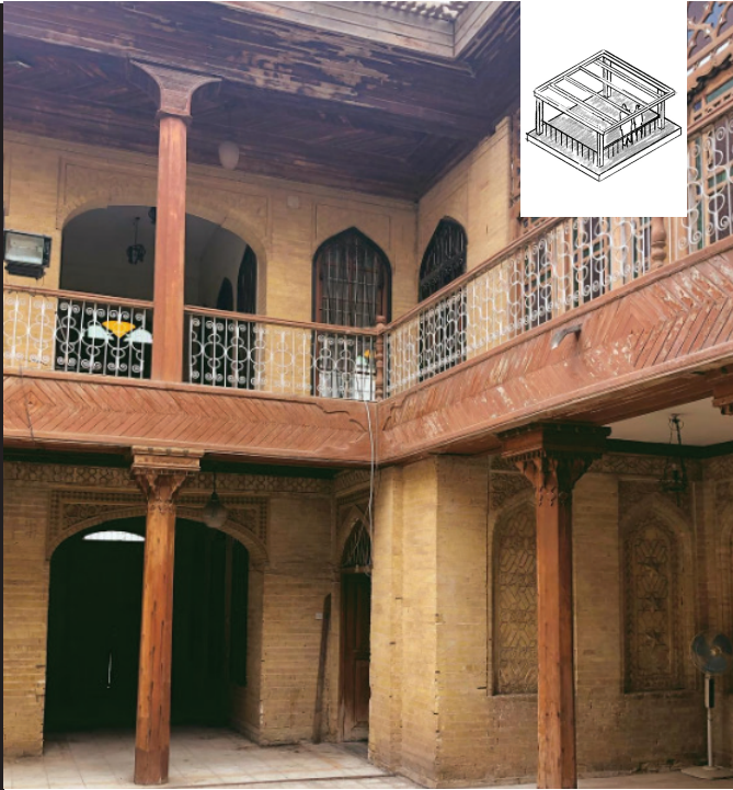
Al-Azzawi (1996) shows that the Baghdadi courtyard house regulates heat through solar gain, radiative cooling, and air movement via the Balgje and Nim / Sardab adapting between day and night cycles.
