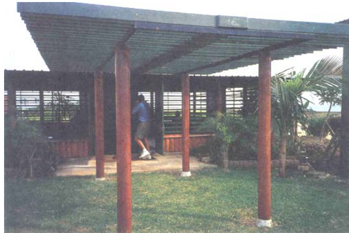
Figure 43. A palm tree used as a column, ending in a 400 mm column every 3.6 m (Source: after Killman & Fink).
