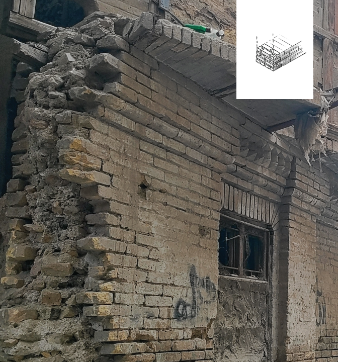
a section of a wall of a Baghdad house, thick with a big thermal resistance
