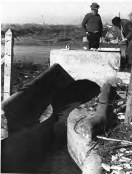
Photo 1. Throatless flume with rounded transition.
