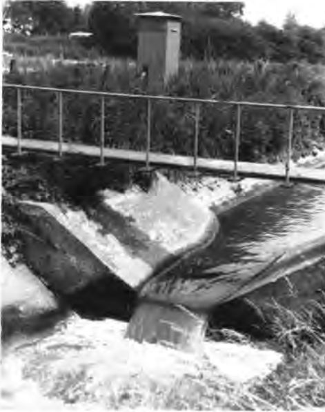
Photo 7. If no kinetic energy needs to be recovered a sudden downstream expansion is adequate.
