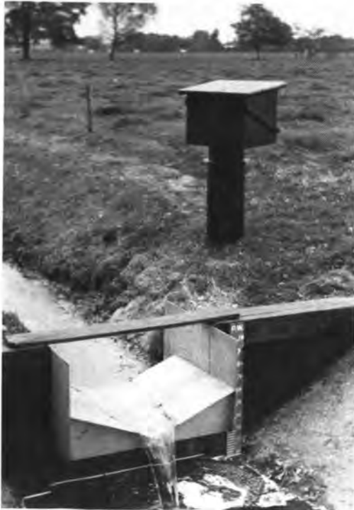
Fig.4.9. Definition sketch for triangular broad-crested weir.
