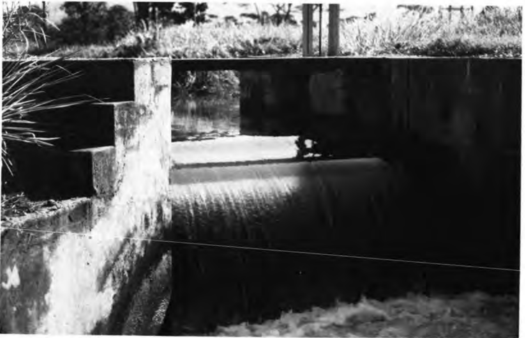
Photo 1. Downstream view of a broad-crested weir.
