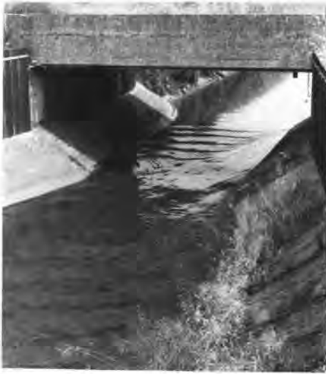
Photo 4. If H_1/L < \text{apr. } 0.08 , undulations may occur in the flume throat.
