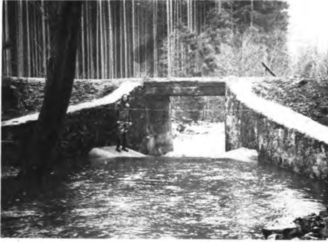
Photo 2. The side walls of the channel in which the weir is placed are not parallel.
