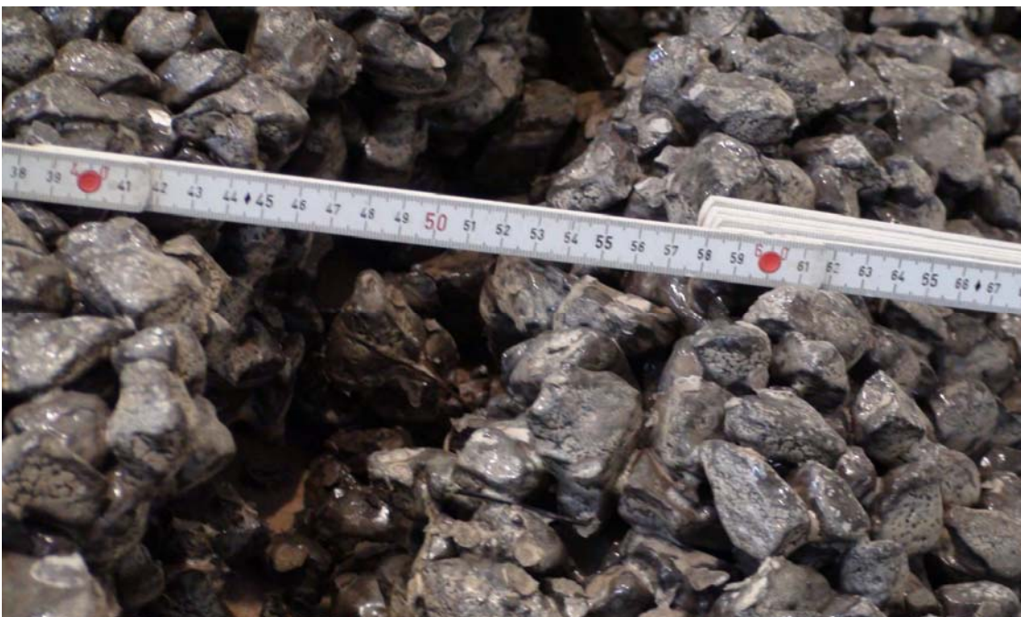
(b) Large gaps in the revetment (breakage)
