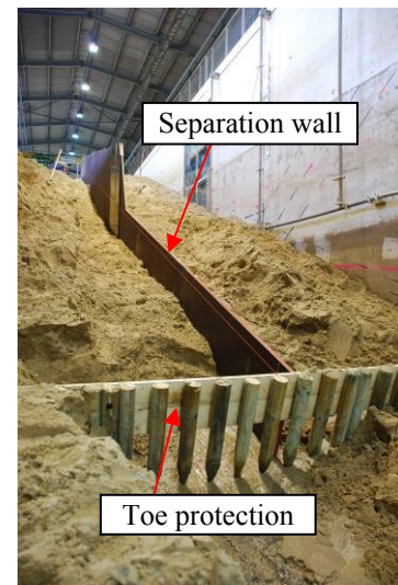
(c) Installed wall with toe
