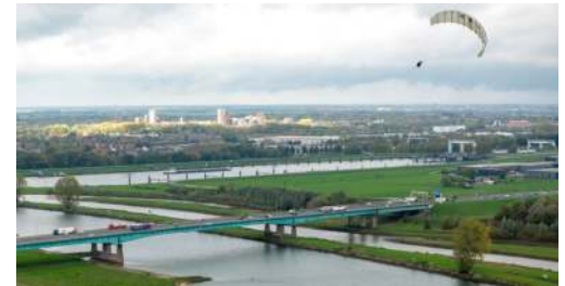
Kitepower in operation near Vianen, the Netherlands, at the Groene Waarden construction site for bridge renovation [1].
