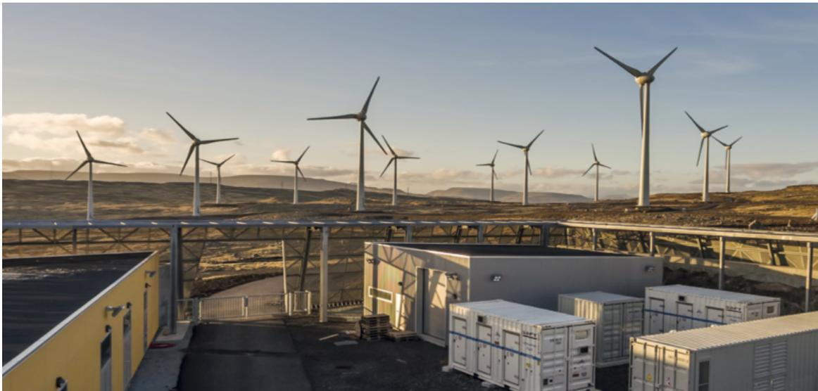
Figure 1.2: Husahagi wind farm - battery system, used for ramping control and ancillary services (EASE, 2017).
