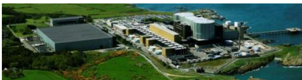
Figure 1: The last Magnox nuclear power station to shutdown at Wylfa, Anglesey, UK [1]
