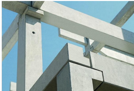
Figure 2.6 Interface between precast members [14]
