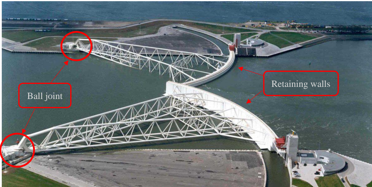
Figure 11: The Maeslant barrier with one arm in sunken mode (the top one in this picture) and one arm in floating mode (the bottom one in this picture). The main purpose of the arms is transmitting the forces, exerted on the retaining walls while closed, to one single joint at the rear of each door. This ball joint gives the doors the opportunity to move freely in three degrees of freedom.
