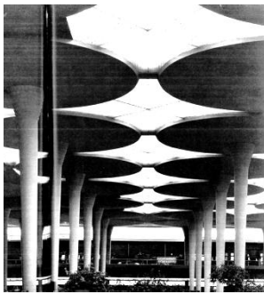
Picture: The loadbearing pillars of the Johnson Wax Factory, designed by F.L.Wright
