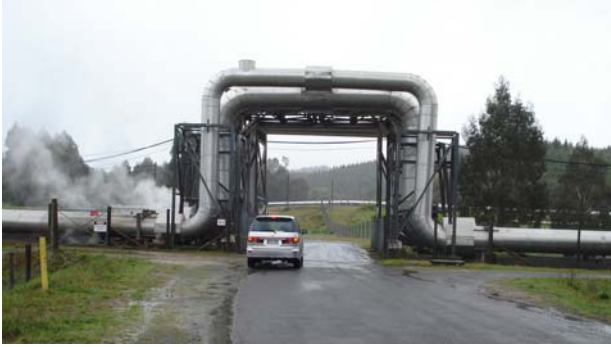
Figure 5 Tertiary road branching off from the Thermal Explorer Highway.
