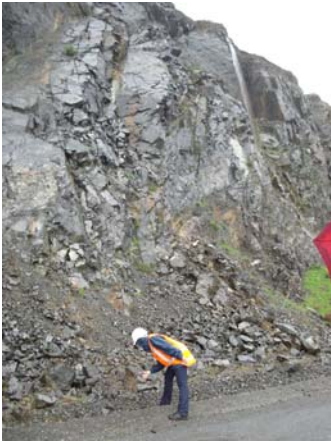
Figure 4 The highly jointed and fractured nature of this rock mass makes it unsuitable as building and cladding stone.
