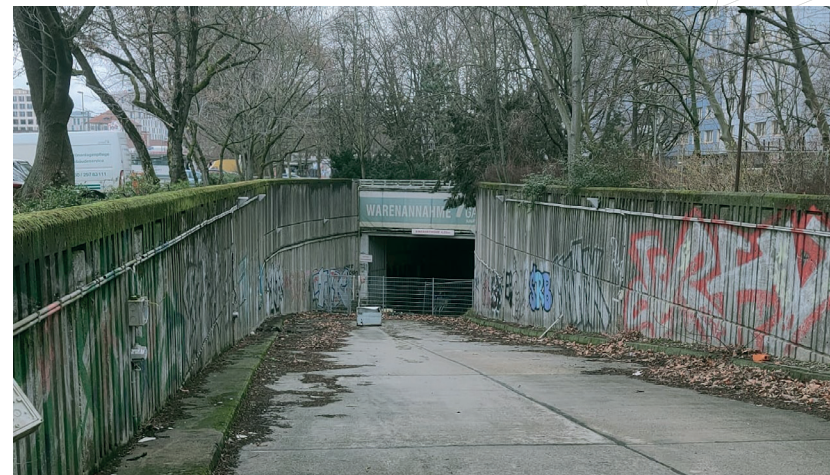
Underground Car Park (out of use)
