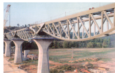
c) Truss steel bridges
