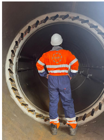
Figure 3.5: HKW jet ring in 2.3m diameter monopile
