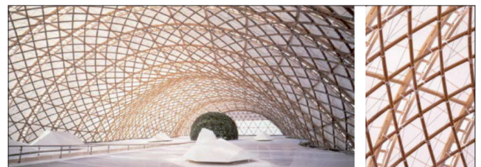
Figure 6. Skeleton of a lightweight structure made of cardboard tubes (Japanese Pavilion, Expo 2000, Hanover, Germany).
