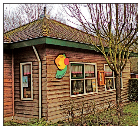
Figure 3. A garden house with walls of unpainted 'red cedar', children's garden De Papaver in Delft, The Netherlands (architect Frank Heyligers, constructed in 1994, photo taken in 2008).
