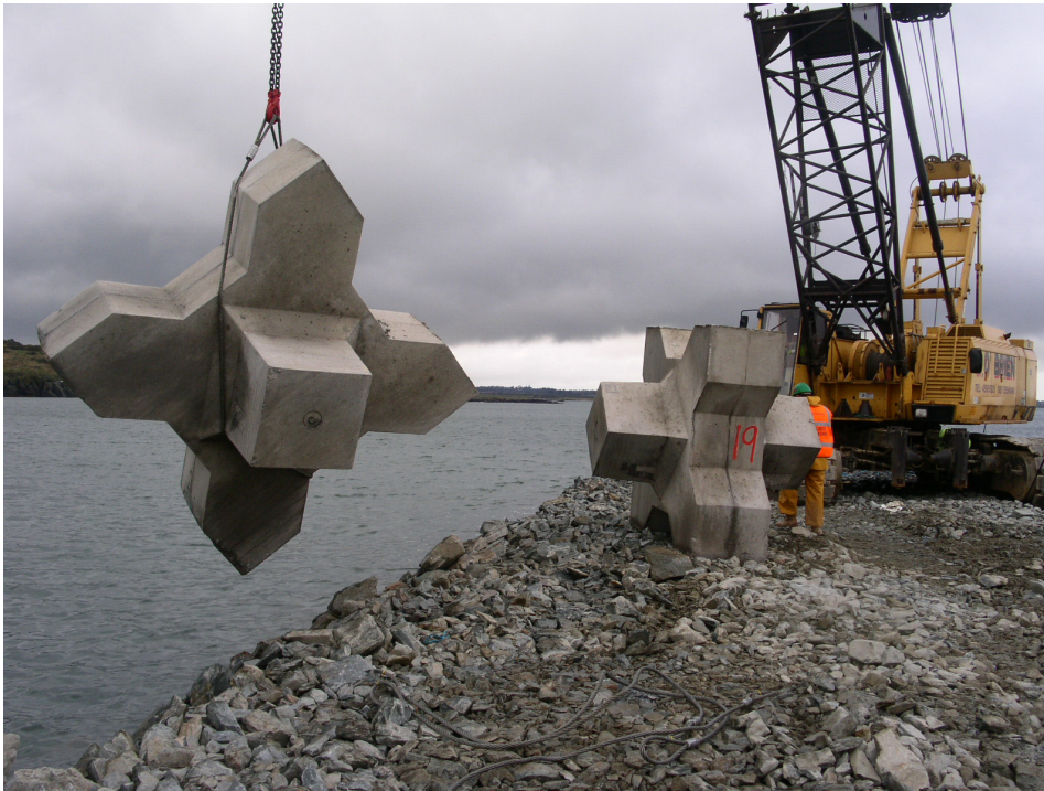
Fig. 2.2 crawler crane with Xbloc attached by sling
