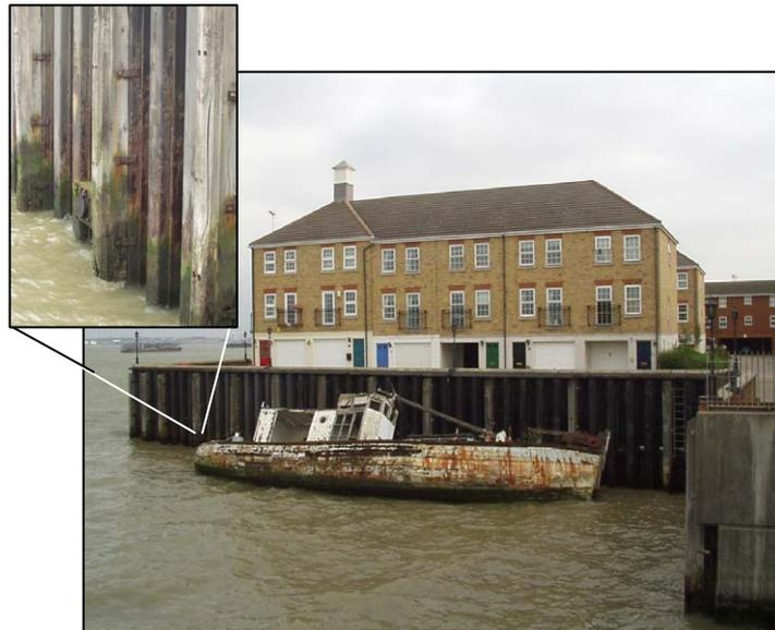
**Figure 3.11. Overview of potential problems with sheet pile walls: 1. ALWC in the splash zone, 2. residential developments have caused 25% of the anchors to fail, 3. the boat left behind disturbs the local loading conditions**
