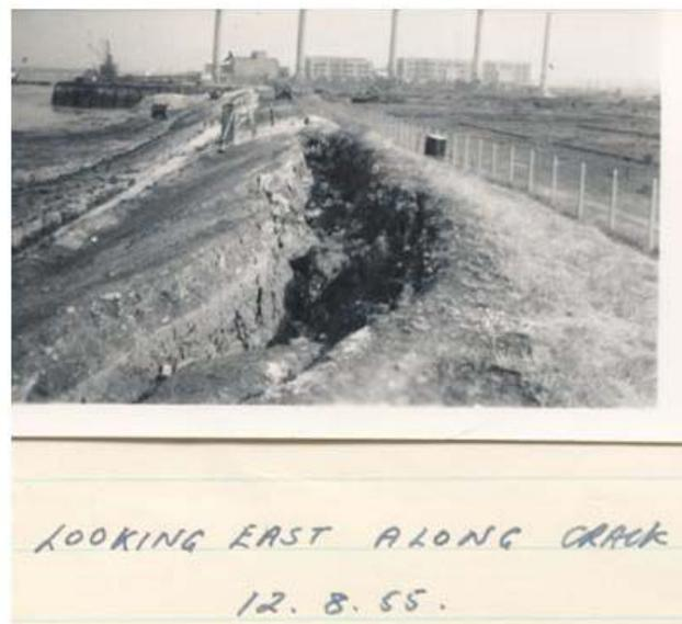
**Figure 3.3.** *Example of a 'crack' in an earth embankment in 1955, with in the background Littlebrook powerstation.*
