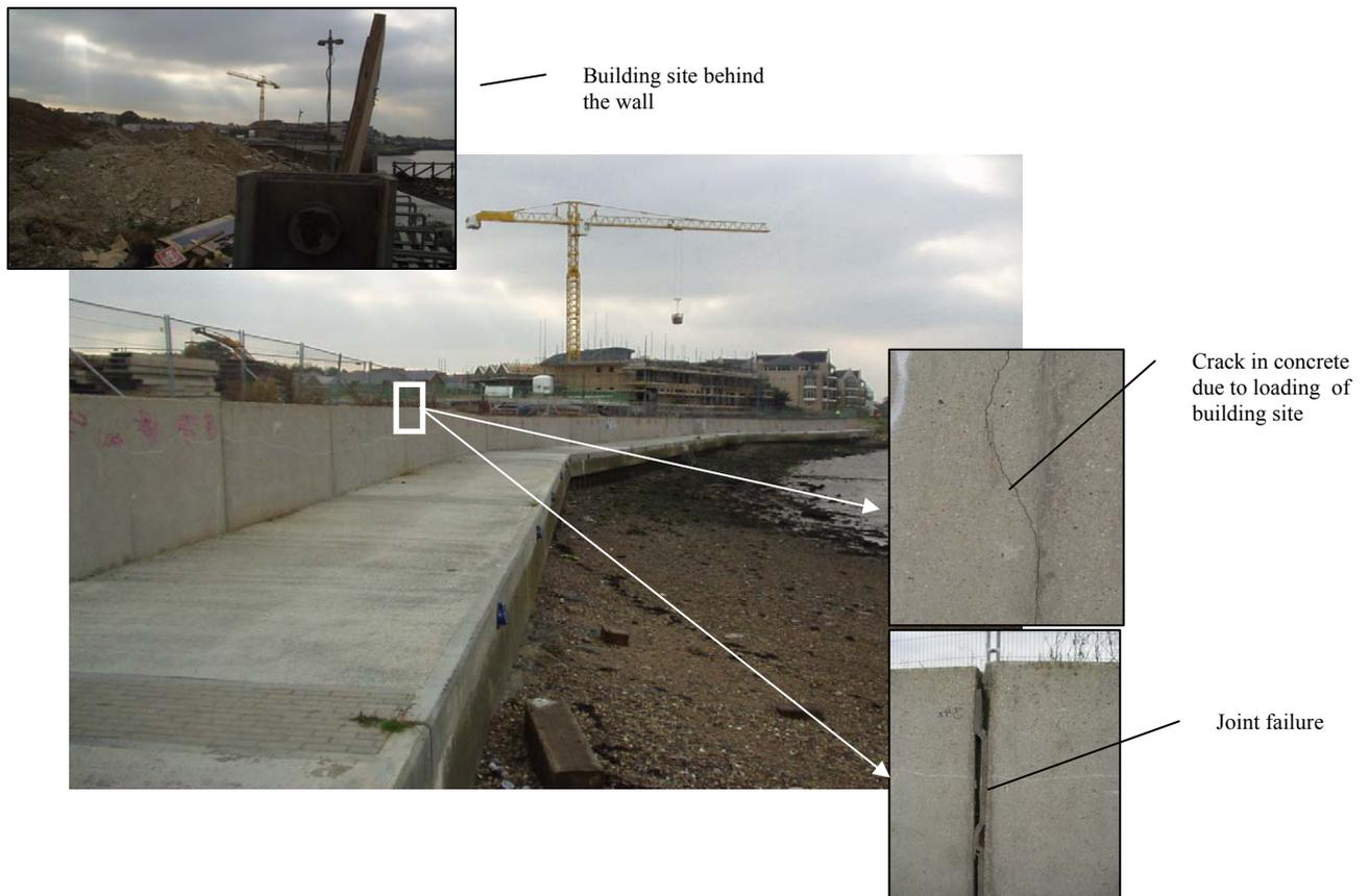
**Figure 3.8.** Impression of damage to concrete wall caused by loading of a building site: 1. cracking of the concrete as the reinforcement is not designed for this type of loading, 2. uneven settlements along the defence line due to the activities on the site behind the wall, 3. joint failure due to uneven settlements / activities
