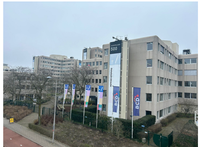
The kanaalcentrum viewed from the south-west (photo: Piet Kerstens)
