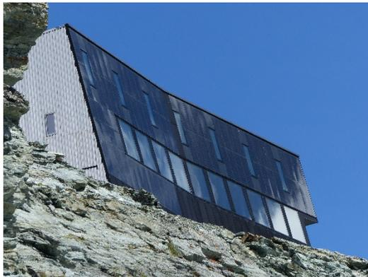
8 CABANE DE TRACUIT - FACADE WITH INTEGRATED PV PANELS AND ENERGY EFFICIENT SHAPE
