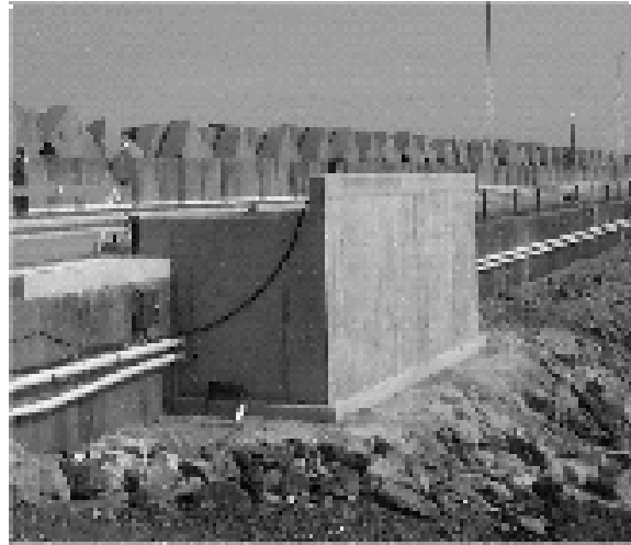
Figure 4: Overtopping container behind crest
