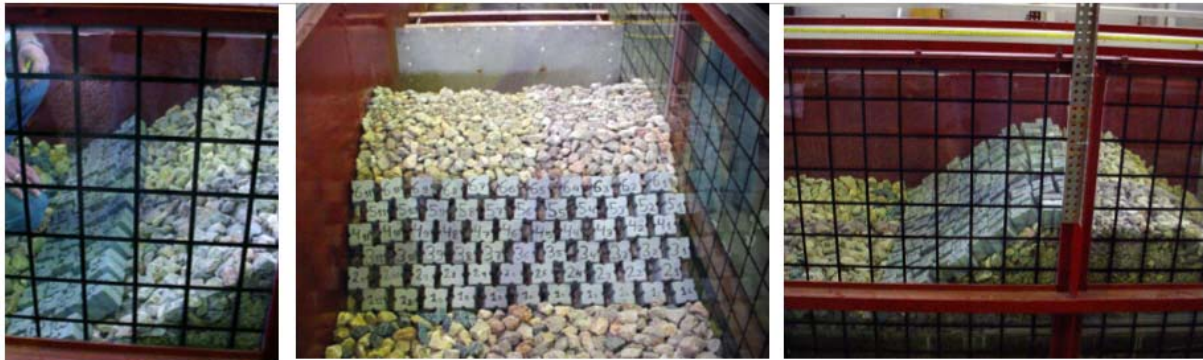
Figure 30: Lower armour layer construction
