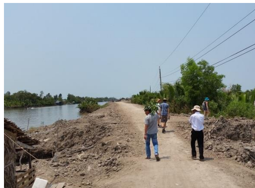
Figure 83: left: road collapsing due to canal bank erosion, right: canal embankment from dredged material.
