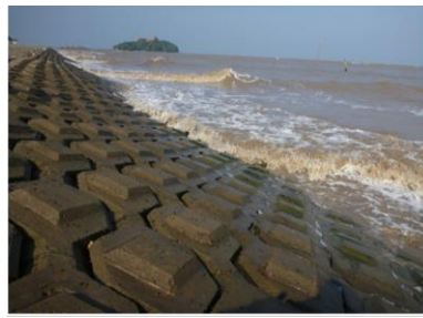
Revetments: placed blocks
