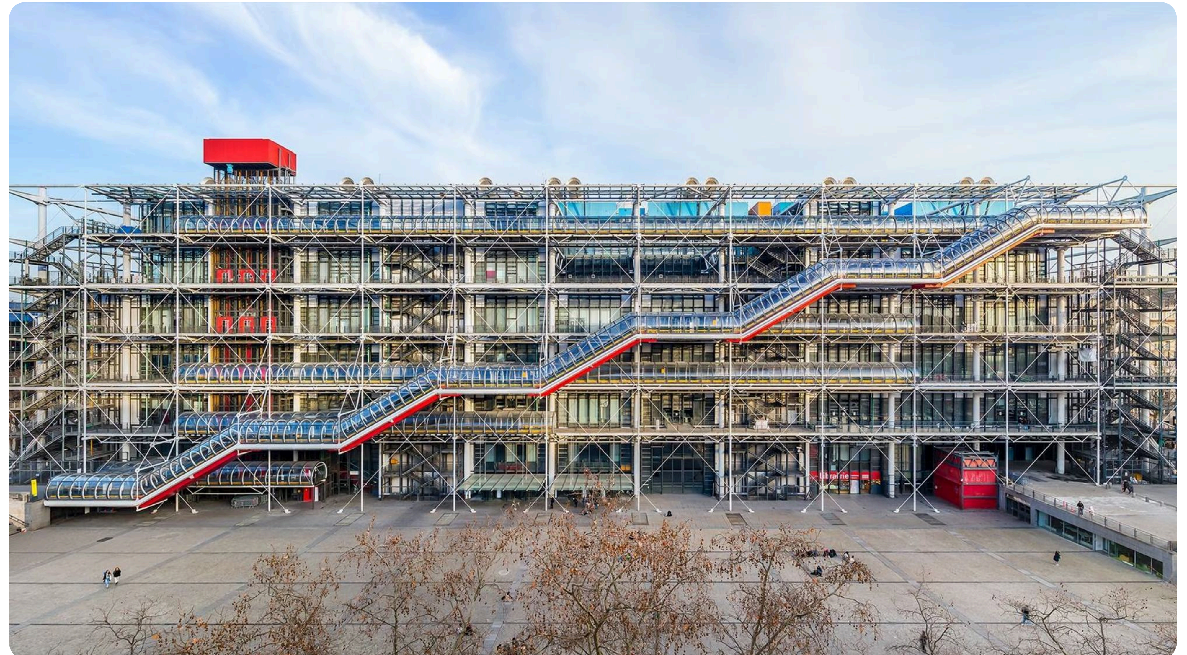
Figure 34 - The Centre Pompidou
