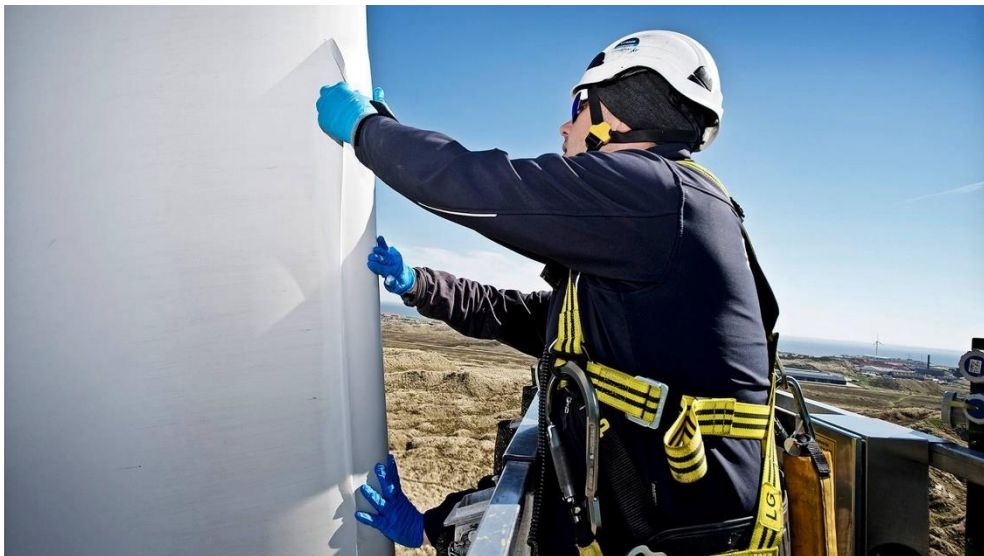
Picture 17. Leading edge protection tape being applied. Image credit: Polytech.com (n.d.).
