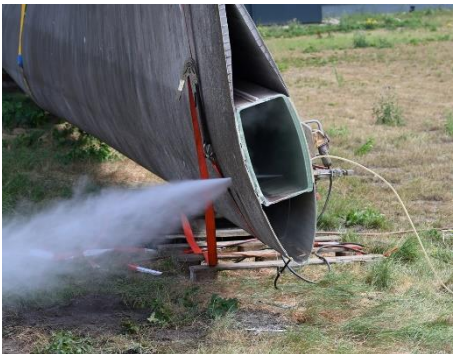
Picture 8. Water jet cutting (Nehls, 2022). Image credit: TNO.
