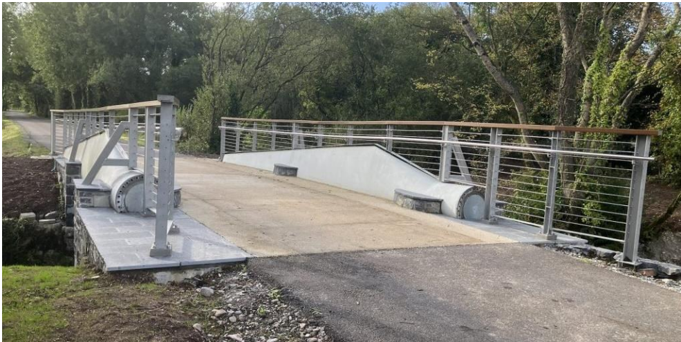
Picture 14. WTB used as structure for a bridge created by bladebridge.ie (2022). Image credit: BladeBridge Repurposing Solutions.
