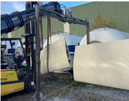
Picture 6. Grinding belt (Ten Busschen et al, 2023). Image credit: Odolphi Technical Support
