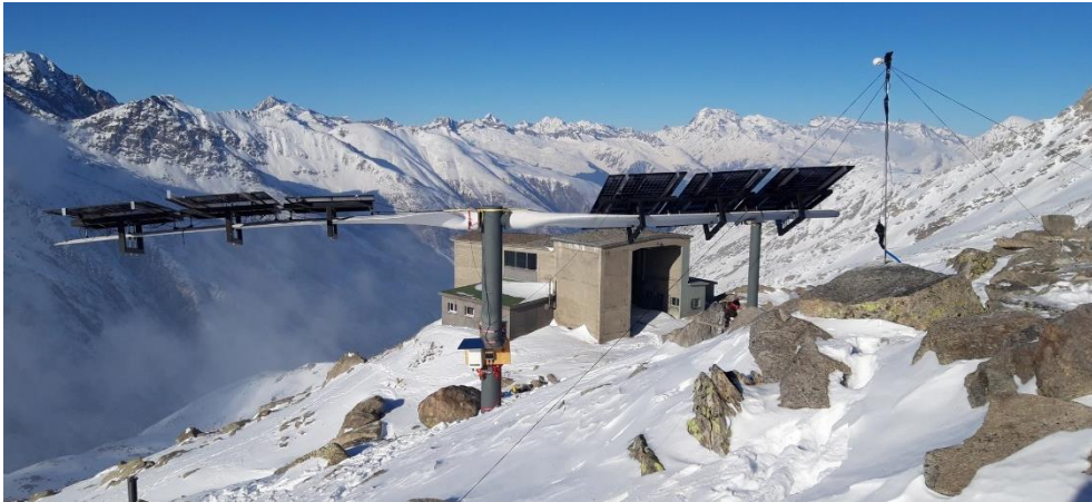
Picture 13. WTB used as structure to hold solar panels created by turn2sun.com (2023). Image credit: Turn2Sun Renewables.
