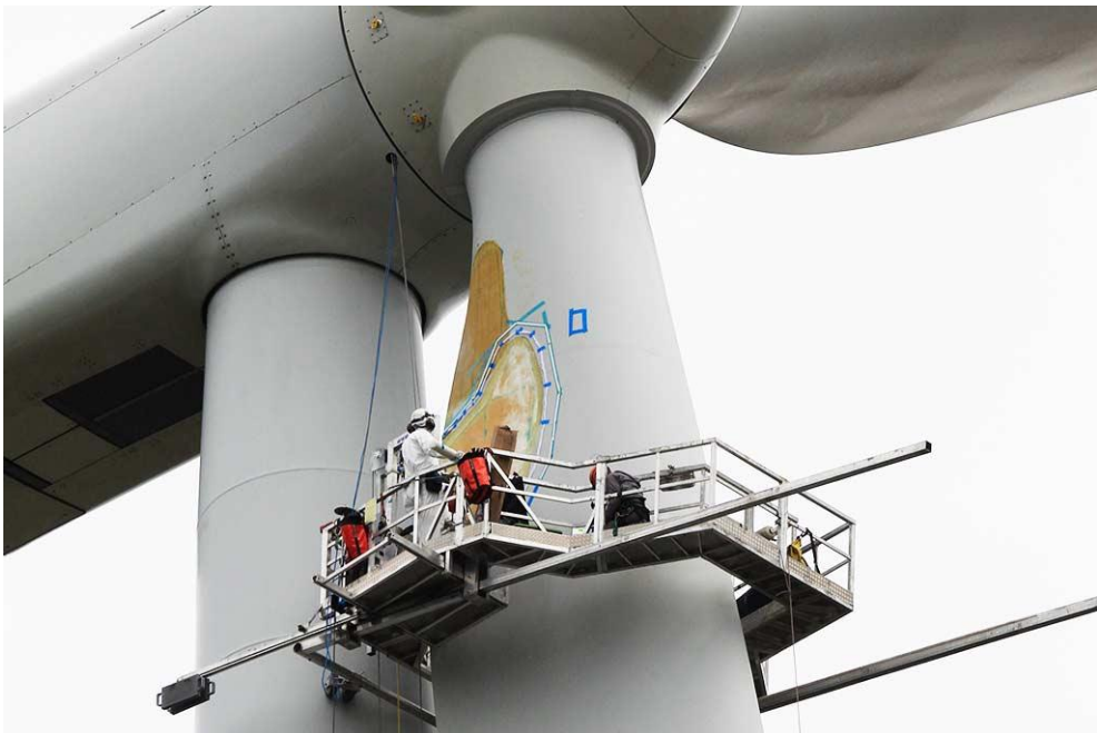
Picture 18. Blade being repaired by ropepartner.com (n.d.). Photo by: J. Castagnetto.
