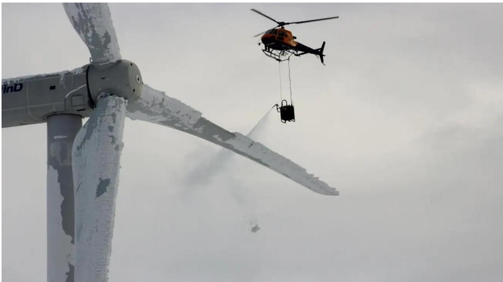
Picture 32. Ice formation on a wind turbine in Sweden, ice is being removed through the use of warm water (Schultz, 2023). Photo credit: Alpine Helicopter Inc.
