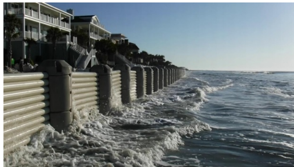
Figure 3.3: Wave dissipation system in front of houses at Isle of Palms (Source: https://www.southcarolinaradionetwork.com )
