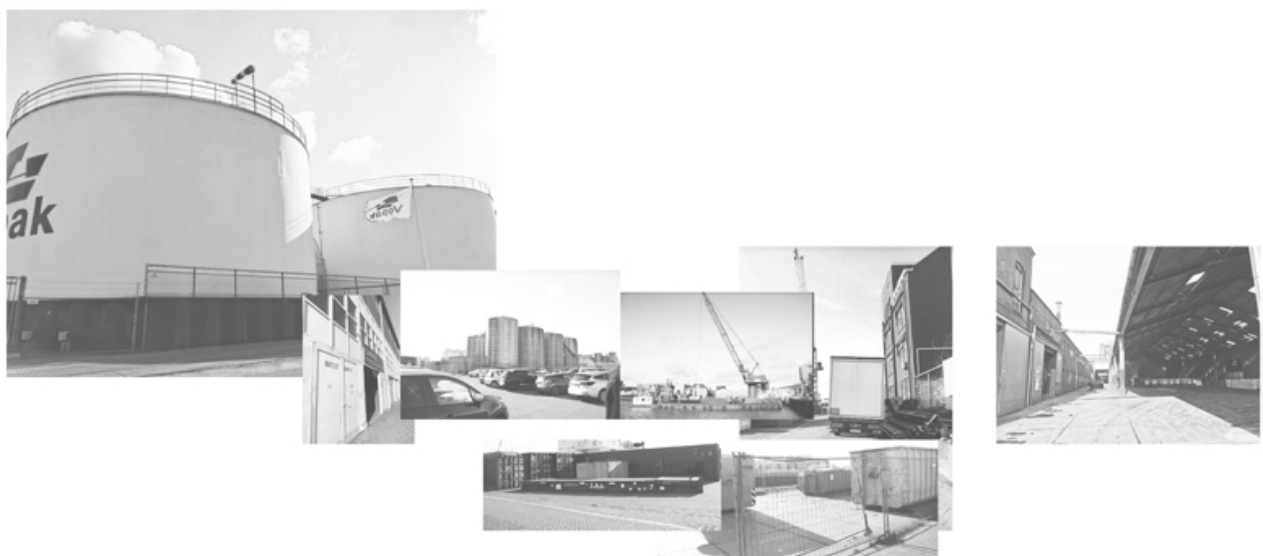
Figure 8: Vokpark: the bio-based distribution center, located in the middle of the Port of Rotterdam
