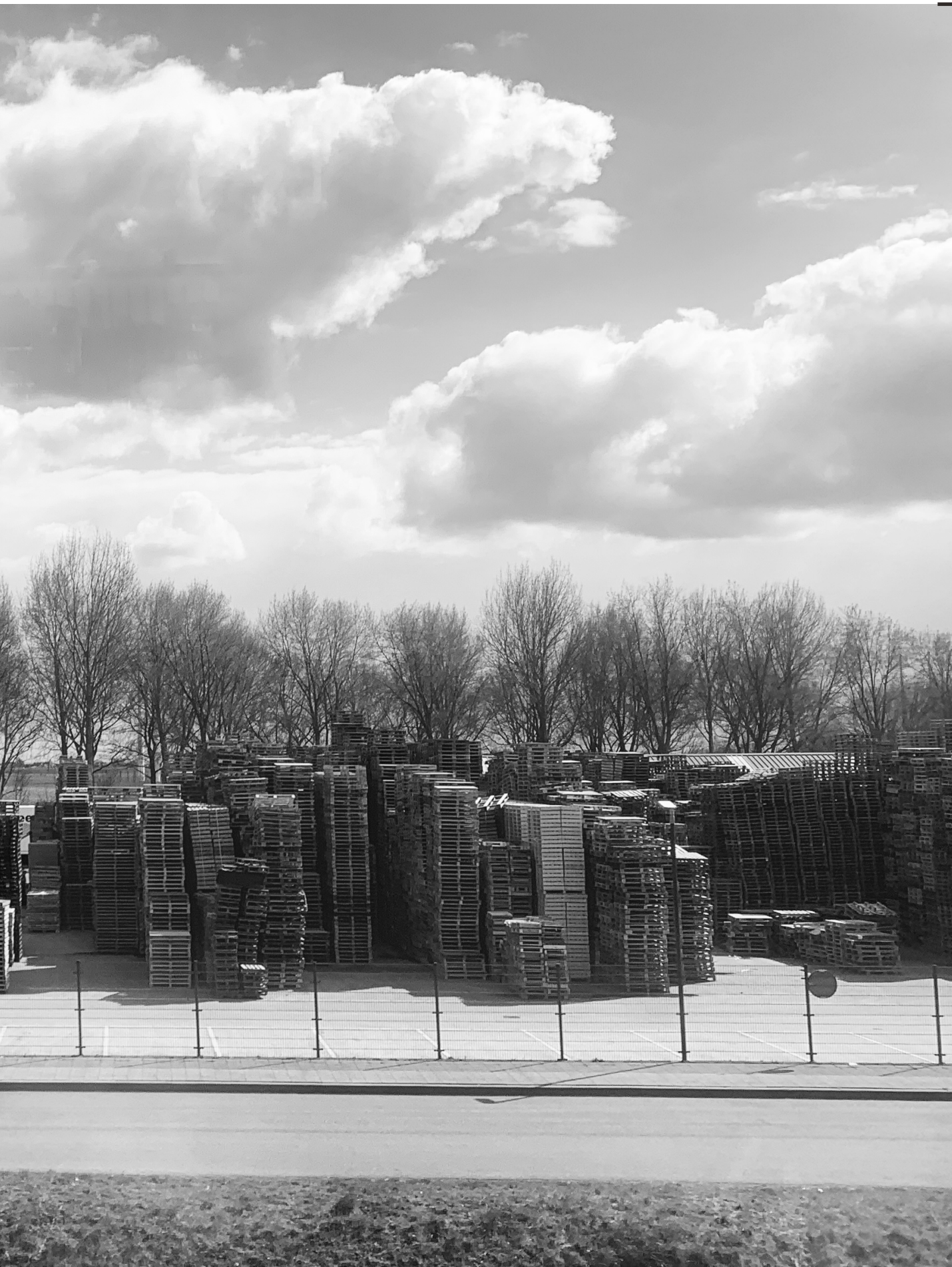
Figure 18: Waste processor facility close to Zoetmeer
