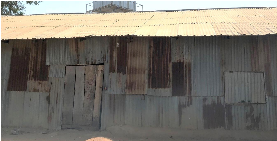
Figure 23: Doors in the camp made from Wooden frames, chicken wire, zinc-coated sheets and wooden planks.
