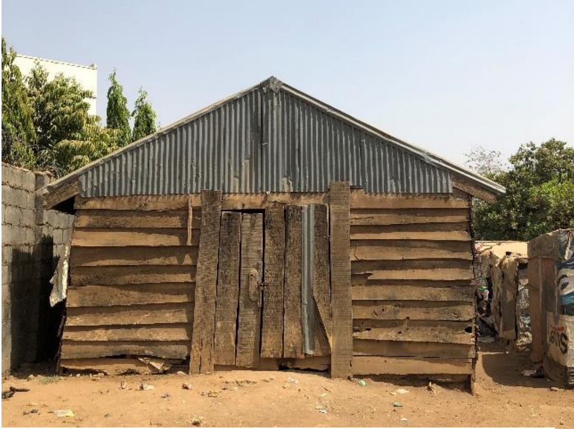
Figure 19: Communal and storage space made out of wood planks and zinc-coated roofing sheets.
