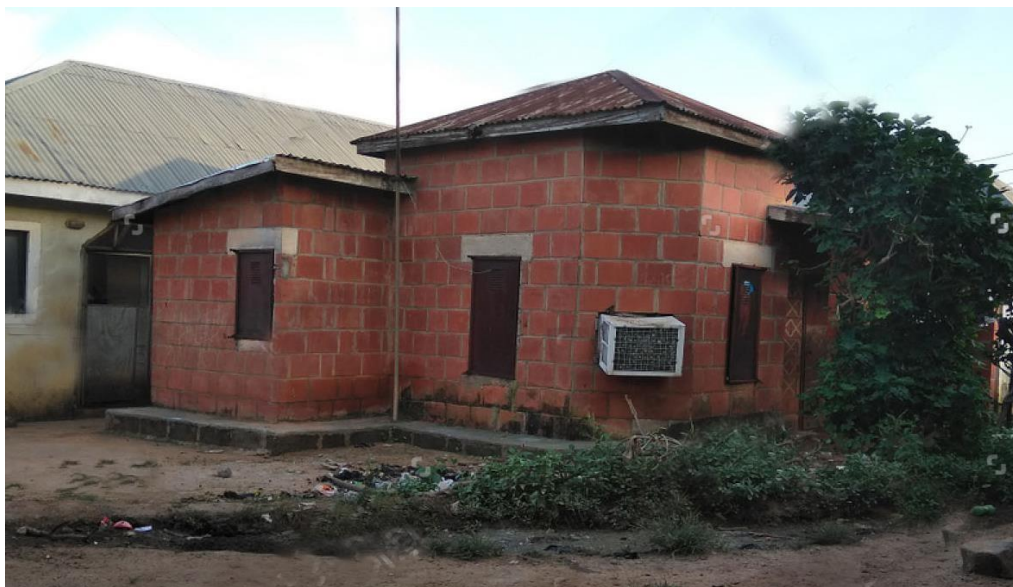
Figure 33: Compressed earth block building Abuja ( https://www.shutterstock.com/nl/image-photo/abuja-brick-house-1228720180 )
