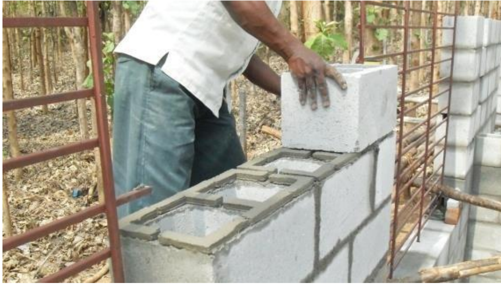
Figure 32: Man laying concrete wall ( https://structville.com/2018/08/how-to-calculate-the-quantity-of-mortar-for-laying-blocks.html )
