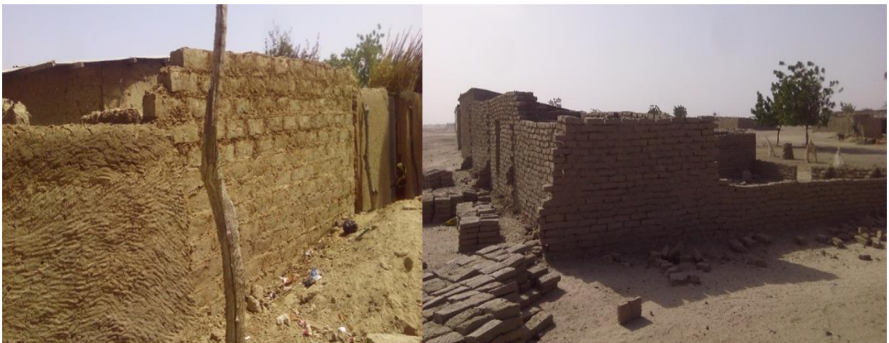
Figure 35: Traditional mud construction Borno (Mercy Corps, 2018).
