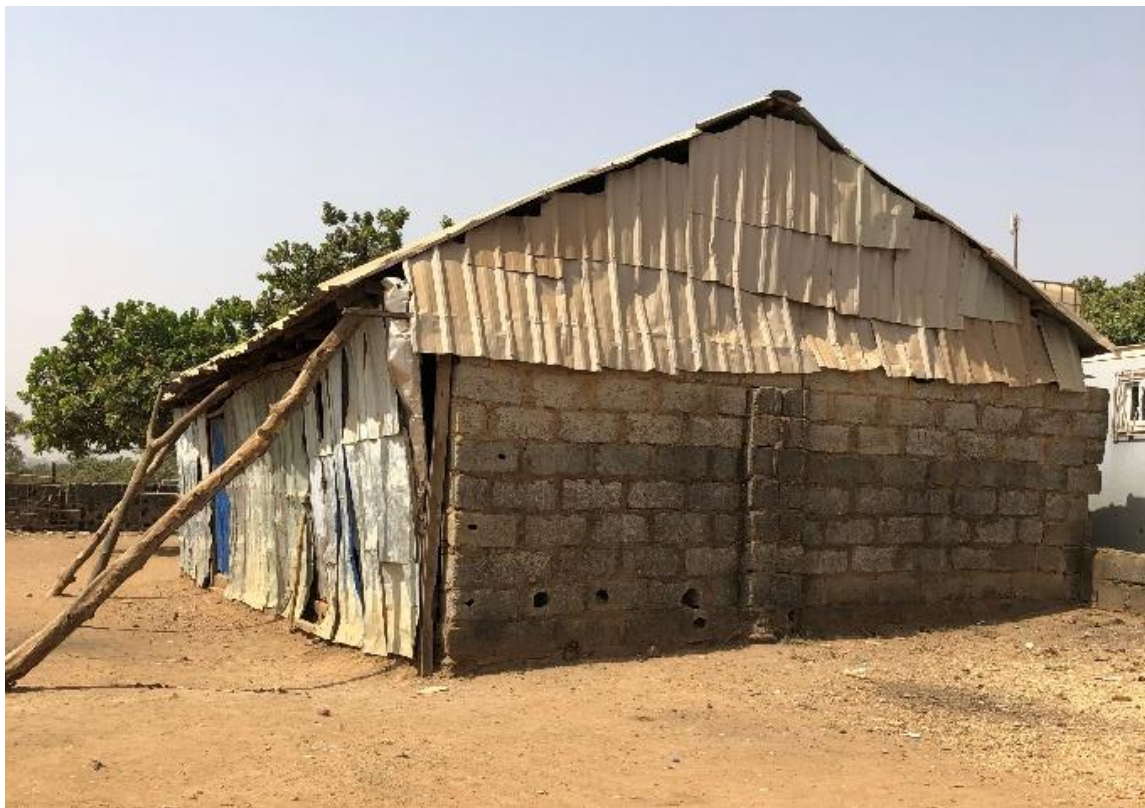
Figure 20: Communal hall made from a combination of wood, roofing sheets and a load-bearing wall.
