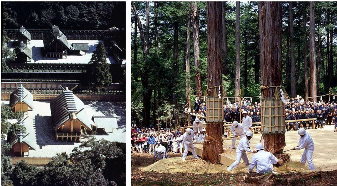
Figures 8, 9 The Shinto Ise Jingu is reconstructed every 20 years using wood from nearby managed forests. The old shrine is torn down and its wood sent around Japan to repair other shrines. Source: Agematsu Tourist Association, 2005.
