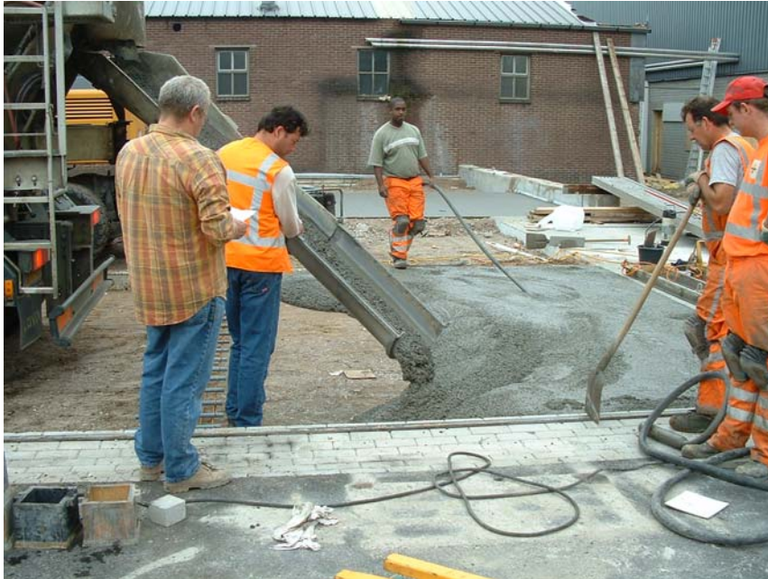
Figure 8.15 Casting and vibrating of the ecological mixture.
