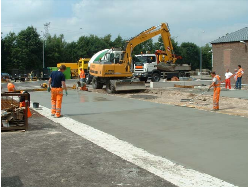
Figure 8.17 Finishing the top surface of the reference mixture.
