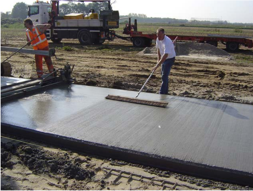
Figure 8.21 The surface is broomed in the transverse direction to create texture and minimize chance of slippage for the users.
