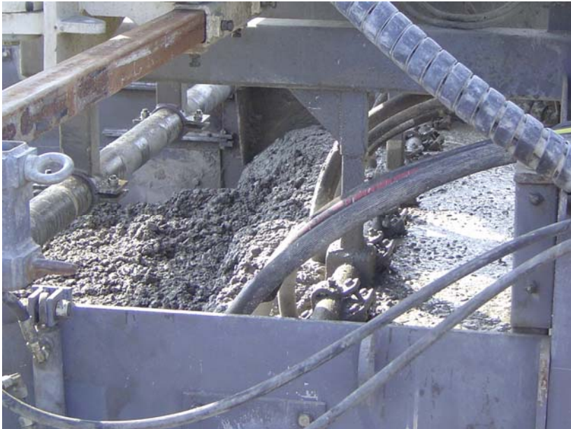
Figure 8.20 Concrete delivered by truck mixer is processed to create a 16 cm thick cycling path.
