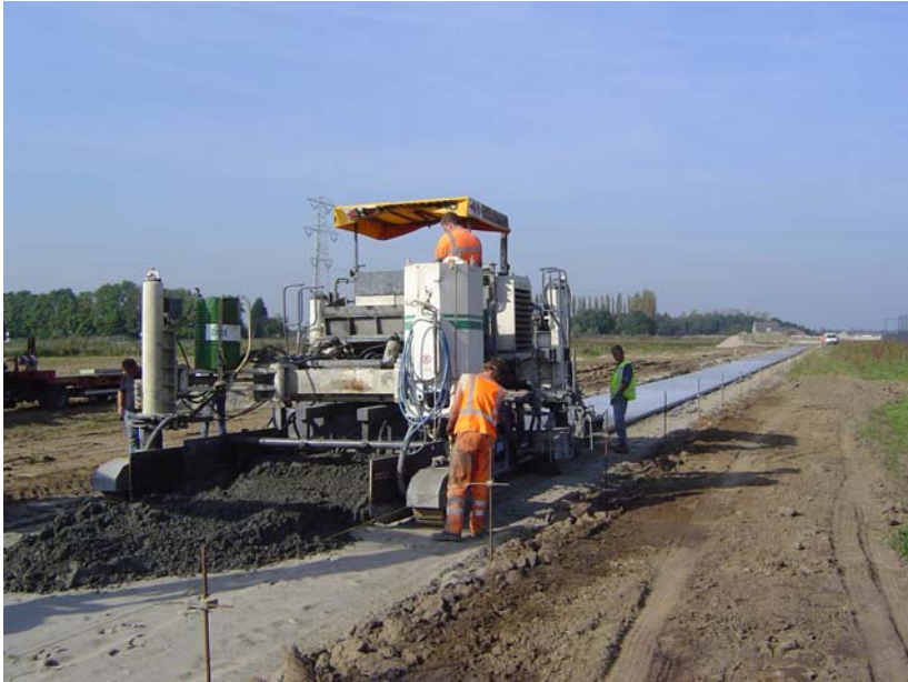
Figure 8.19 Production of cycling path Rosmalen by slipform paver.
