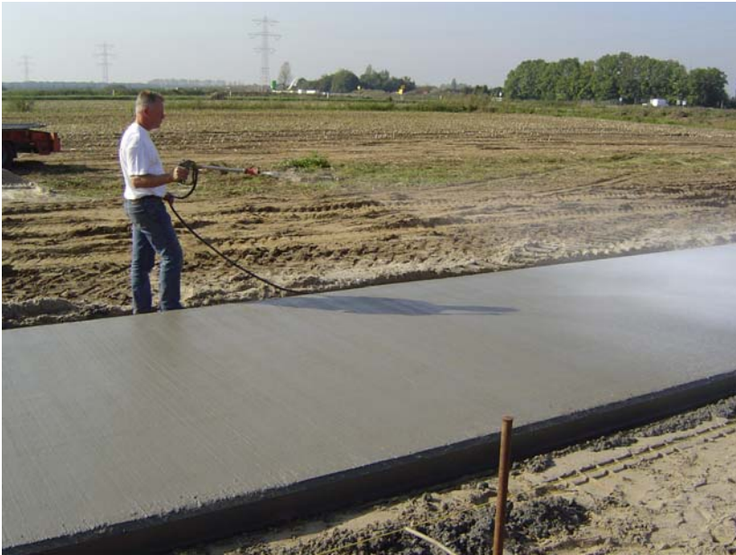
Figure 8.22 Spraying of the curing compound to prevent drying out at early age.
