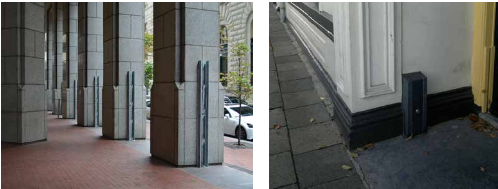
FIGURE 4.10 Example of retrofitting dry proofing to an existing office building in Manhattan, New York (left) and an historical building in Kampen, The Netherlands (right). Both dry proofing solutions are based on installing panelised flood protection during high water conditions. Photos by author.
