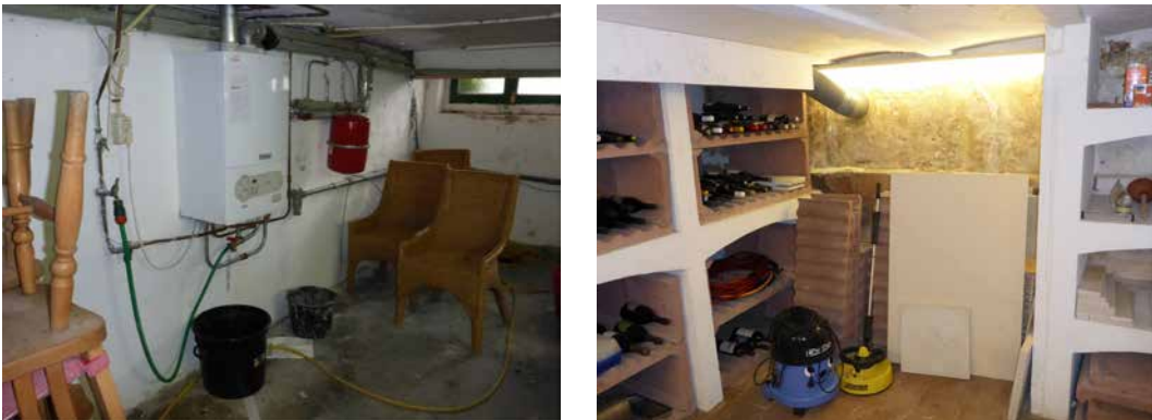
FIGURE 6.4 A substantial part of the costs of flooding of residential buildings is due to the vulnerability of building systems, interior and storage of sensitive goods in basements. Photos: Kuijk & Boer (2015).
