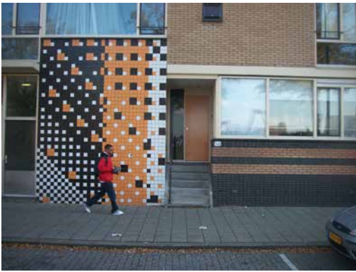
FIGURE 4.11 Dry-proofed architecture in Feijenoord, Rotterdam. The blank walls of dry-proofed buildings may have a negative visual effect on the streetscape and require careful design. Photos by author.
