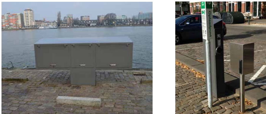
FIGURE 4.15 Elevated shore power supply facility in Dordrecht, The Netherlands (left) and flood protected power distribution station at the Noordereiland, The Netherlands. Photos by author.
