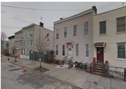
FIGURE 7.6 Typical Red Hook building with semi below grade basement and ground floor apartment located below the Base Flood Elevation (BFE). Photo: Google StreetView.
