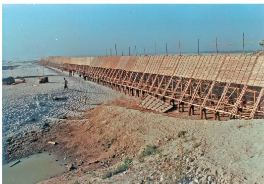
Figure A.1: Bandal structure constructed in the Brahmaputra-Jamuna, adopted from (Mosselman, 2006)
