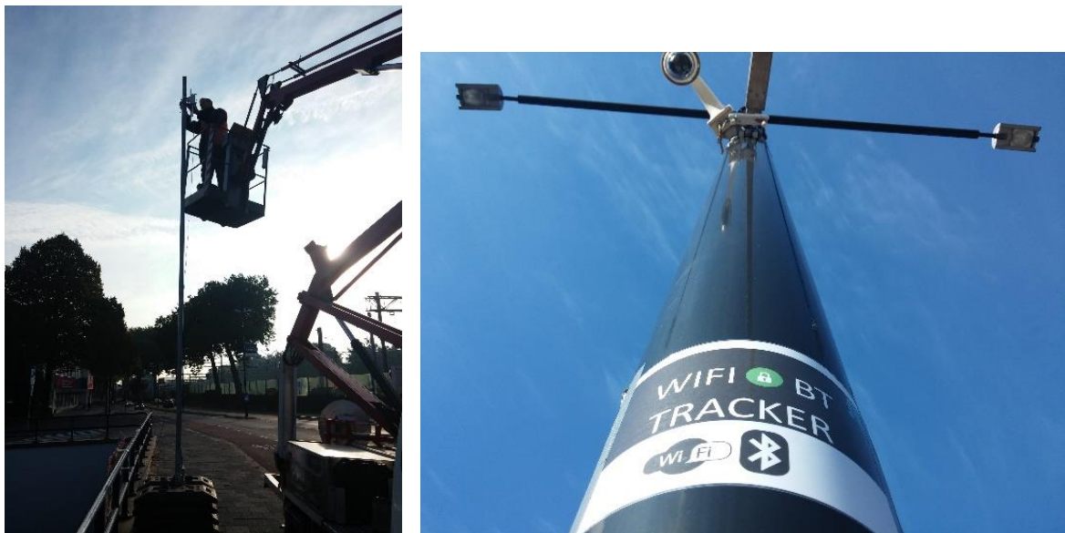
Figure 8: Wi-Fi sensor placement in the research area in cooperation with the technical department of the Municipality (left) and notification signs informing people about their existence (right)
